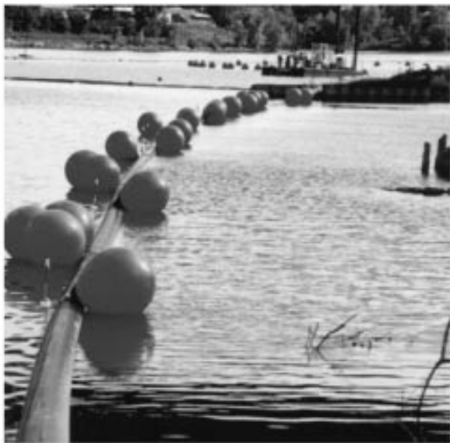
A silt curtain prevents sediment from moving downstream during the dredging operation at SMU 56/57.
