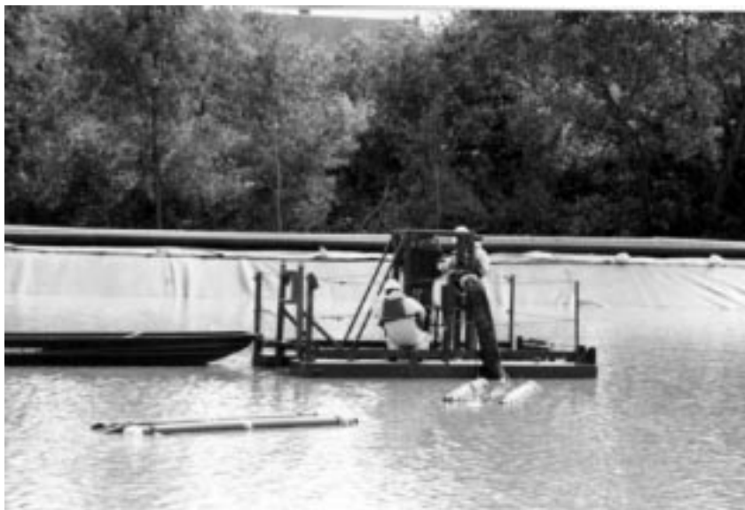
Crews remove contaminated sediment in 1999 from dewatering lagoon at SMU 56/57 near Green Bay. Sediment removal will resume this summer under a Federal agreement.
